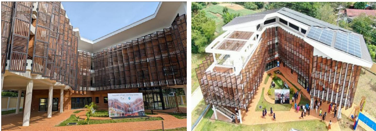
Figure 4: Showing building form and solar features of a nearly zero-energy building (nZEB), Accra. (Source: Energy Commission Ghana, n.d.)
